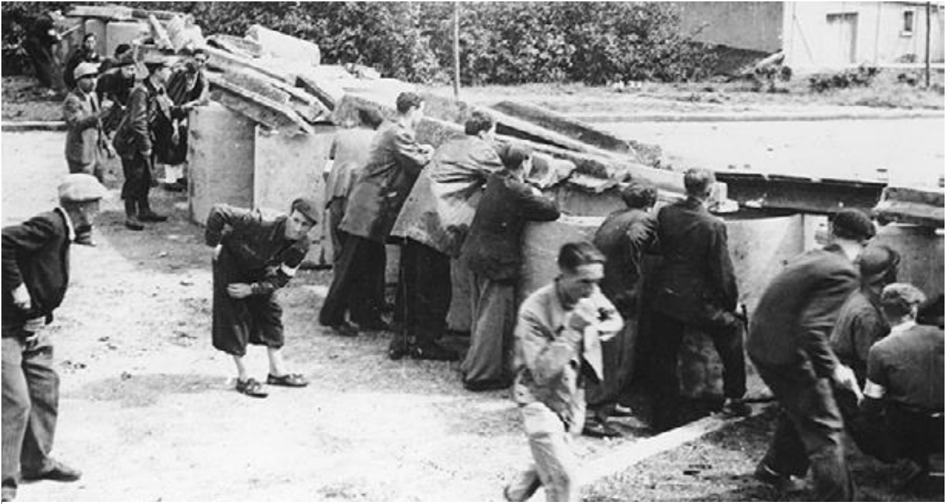
Fig. 8: Prefabricated modules make assembly faster and easier.
